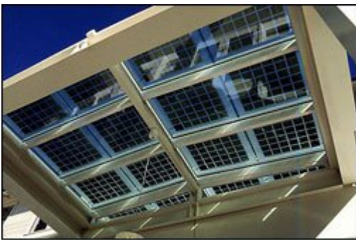
A PV skylight entryway (Courtesy of DOE/NREL)
